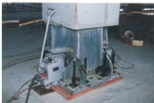
Jacking up a pillar of the passenger Terminal Building
